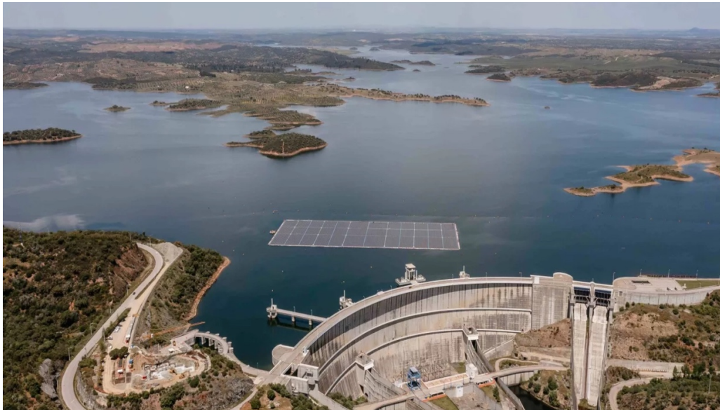
Fig. 1.5: The first hybrid FPV–hydropower system, established in 2017
